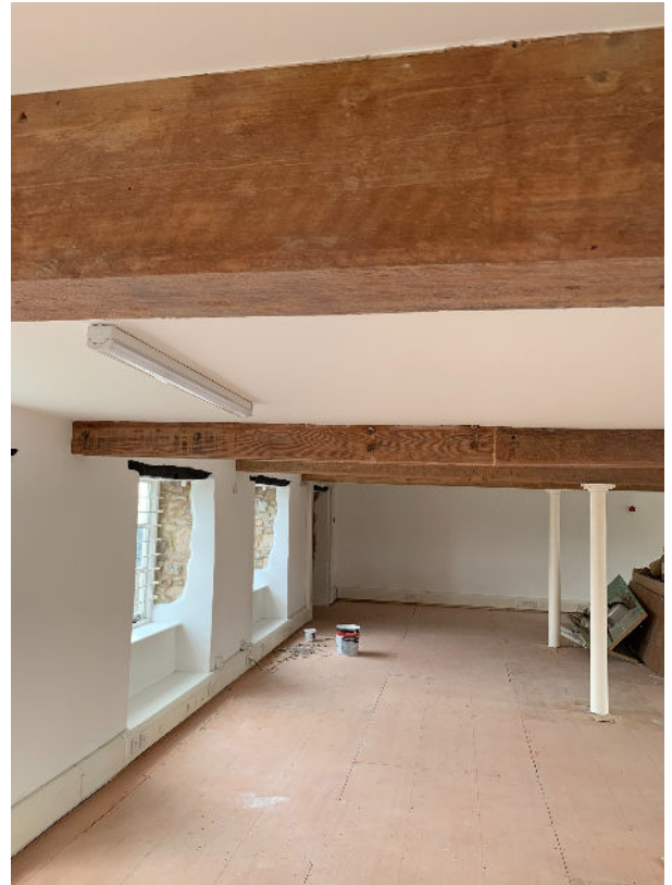
The Bone Mill, Charfield - protection to timber and structural steel in a historic building.
