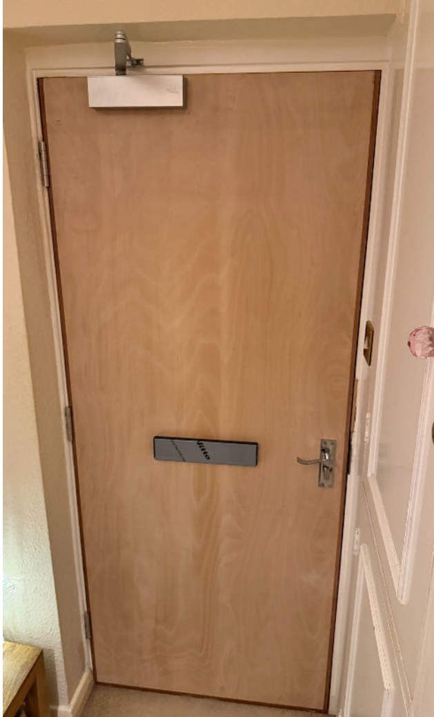
Withyolt Court, Cheltenham - new FD30 fire doorset photographed during installation.
