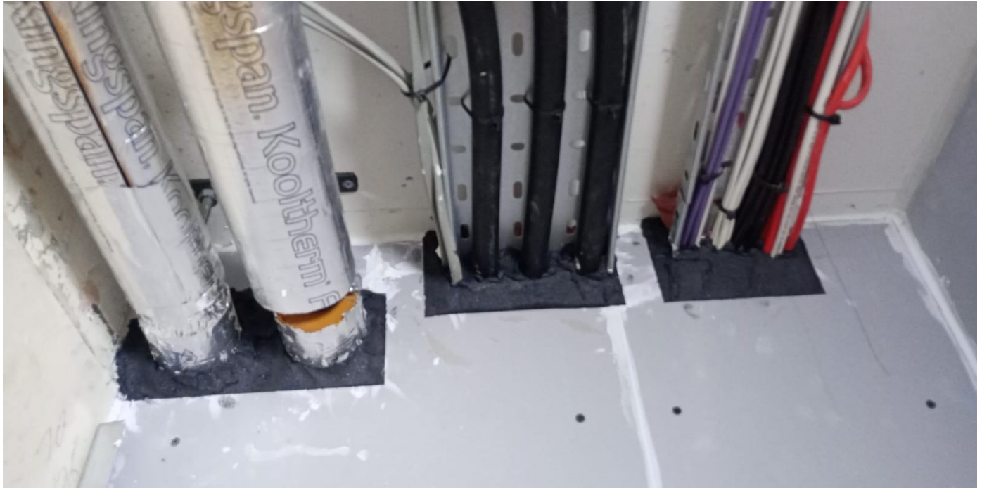
Oriel House, Cheltenham - fire-stopping to service penetrations within riser cupboards.
