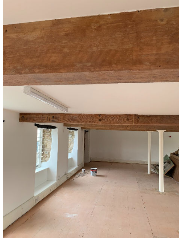
The Bone Mill, Charfield - protection to timber and structural steel in a historic building.
